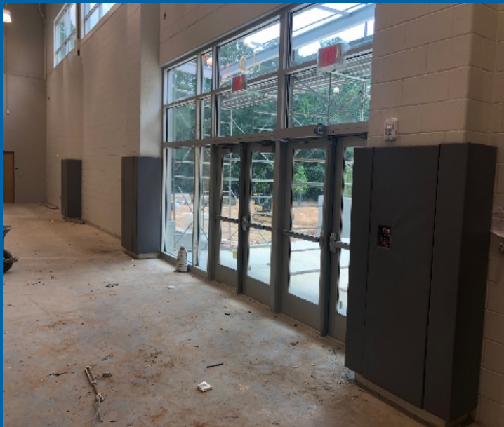
Gymnasium Wall Pad Installation
