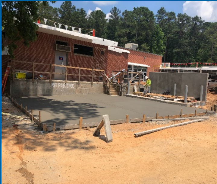
Loading Dock / Dumpster Pad Concrete
