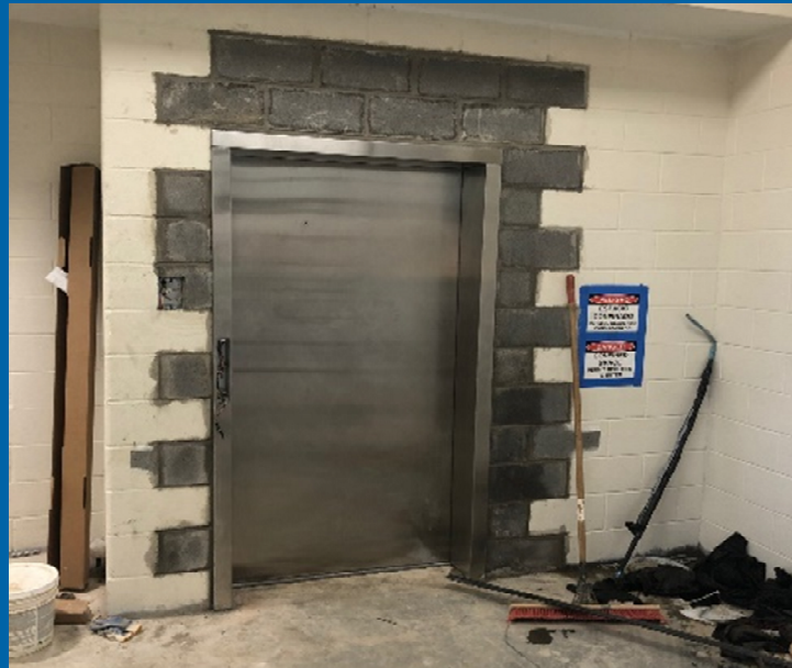
Elevator Installation and CMU Infill
